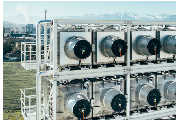
Image depicts a Direct Air Capture system. (Photo: Climeworks)
