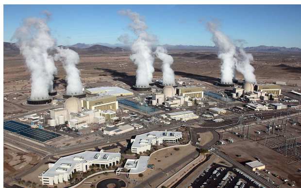
Image depicts the Palo Verde Nuclear Generating Station – one of the United States' largest power producers for nearly 30 years – all of it clean and carbon-free. The plant is a critical asset to the Southwest US, generating more than 32 million megawatt-hours annually – enough power for more than 4 million homes and businesses. (Photo: Business Wire)
