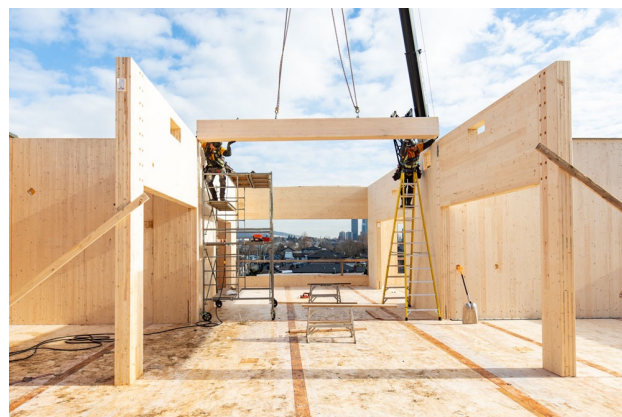
Image depicts a building being constructed using mass timber. (Photo: naturally:wood)
